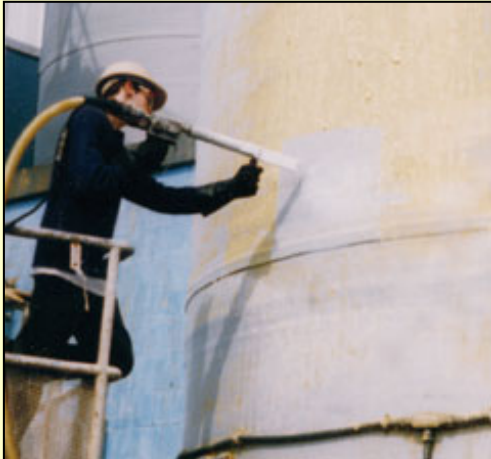
Dry ice cleaning of fiberglass silo
